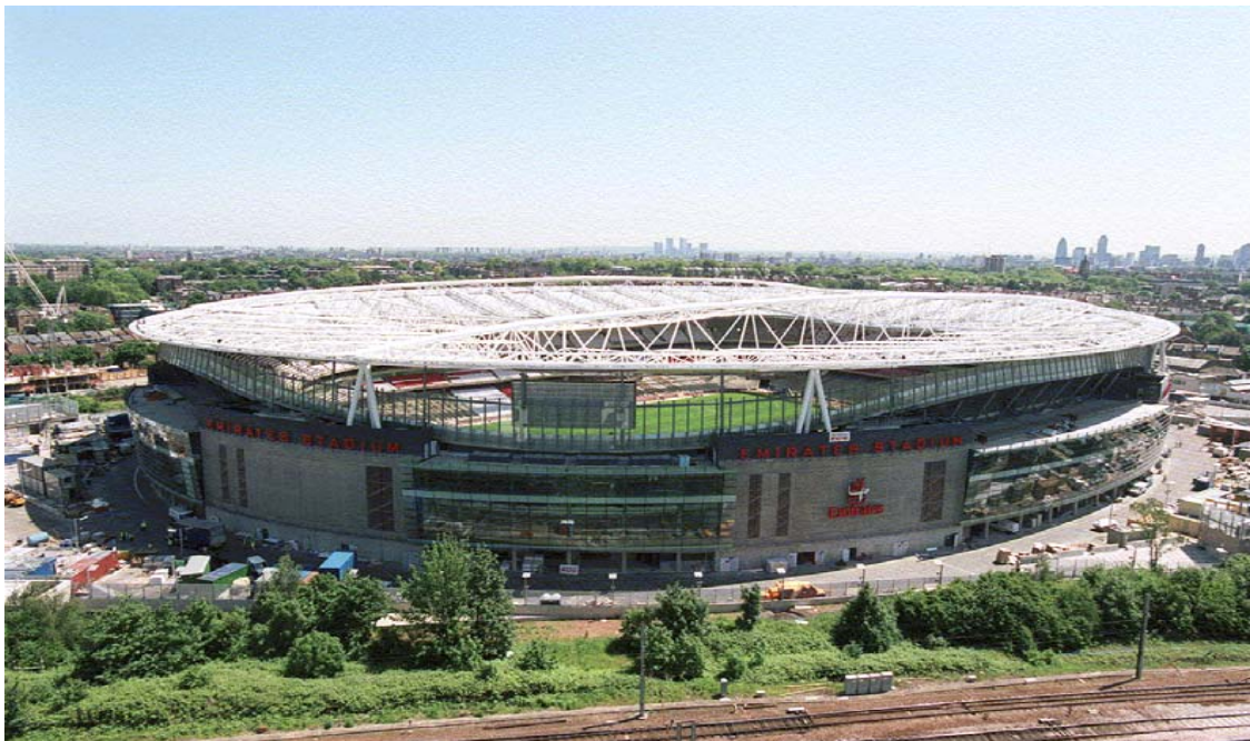
Date of picture: June 2006
